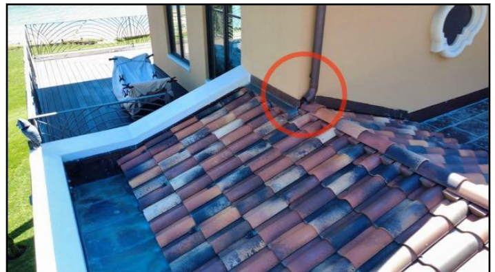
Discharge onto roofs
