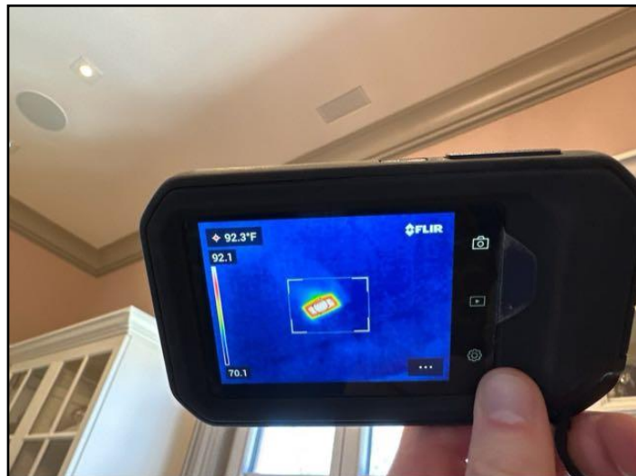
General view of heating system
