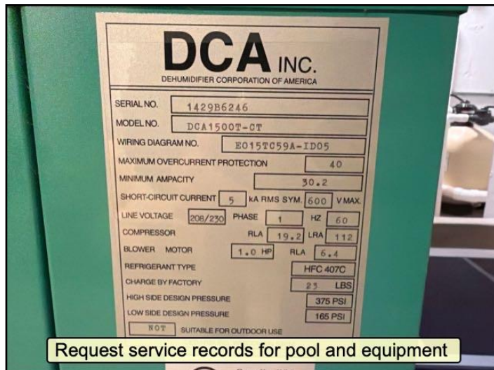
General view of pool and equipment
