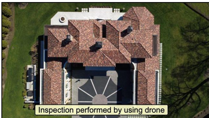
Roof inspected - drone
