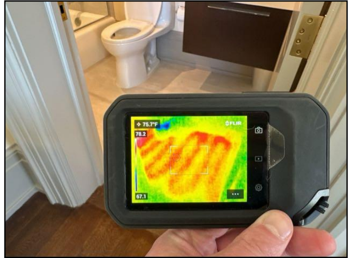
Hot water radiant piping
