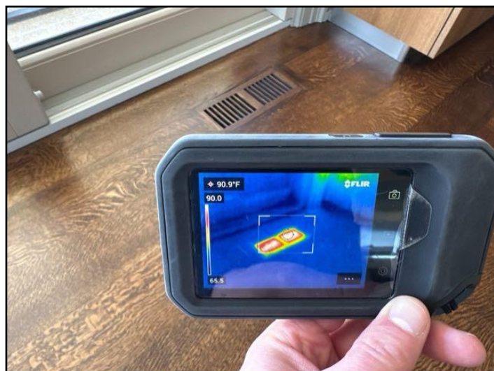
General view of heating system
