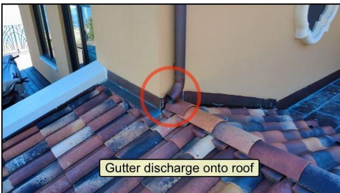
Discharge onto roofs
