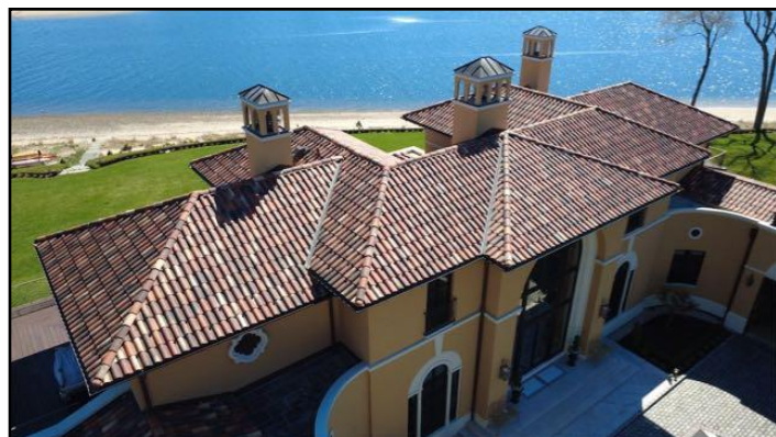
Roof inspected - drone
