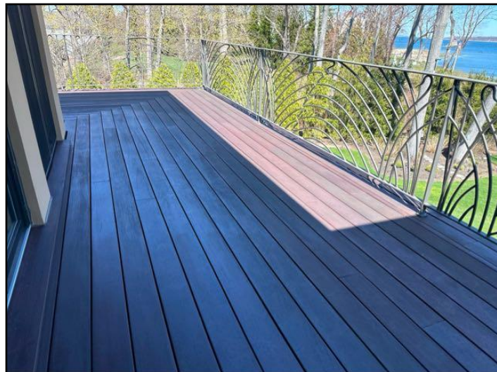
Deck covering roof
