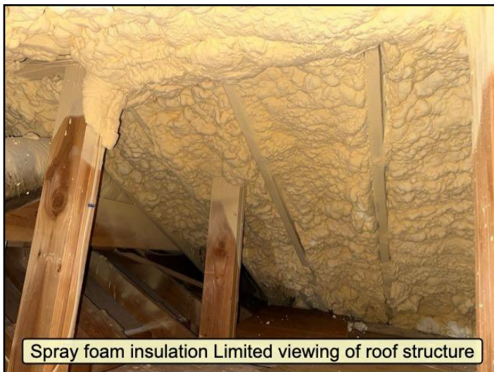
Insulation limited viewing of structure
