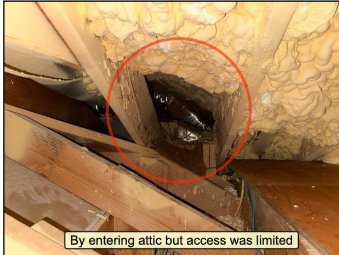
By entering attic, but access was limited
