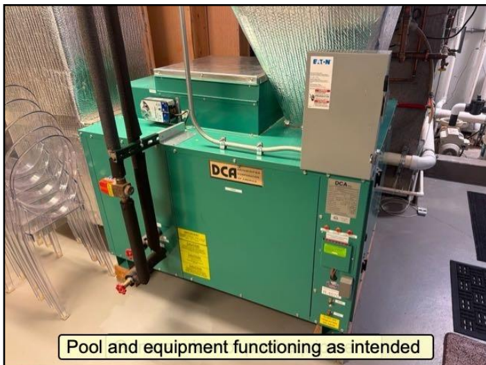
General view of pool and equipment
