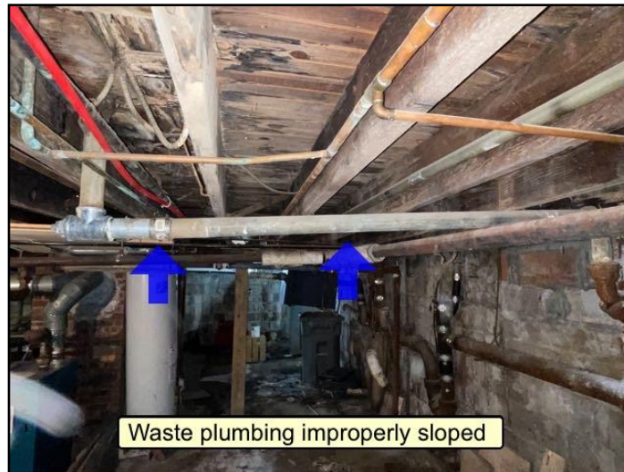
Poor slope
