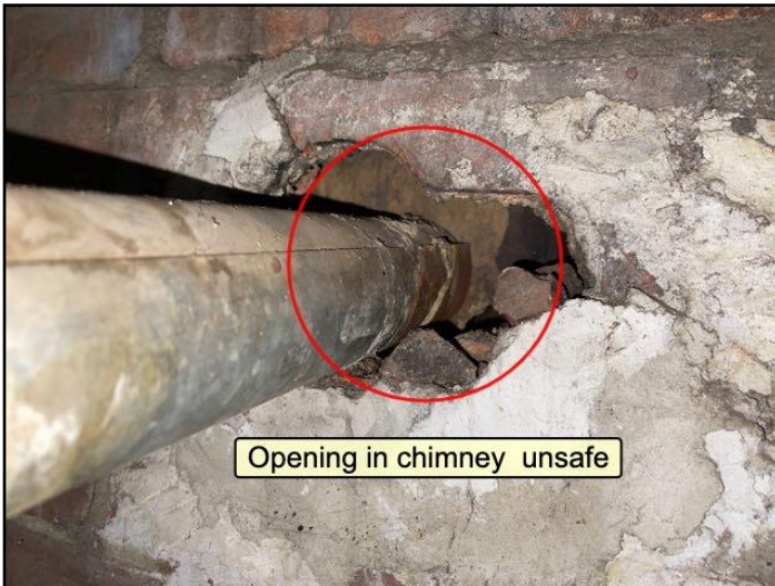
Poor connections
