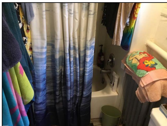
Bathroom in need of upgrading. Recommend...
