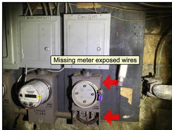
Unprotected openings
