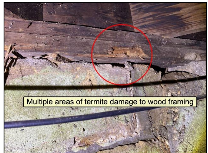
Termite damage
