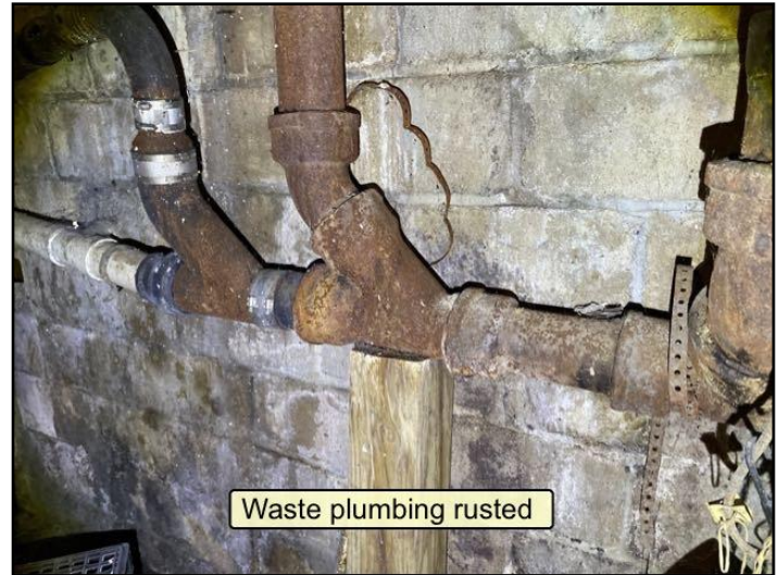
Split, rusted or damaged
