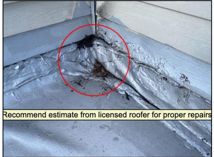
Licensed Roofing Contractor
