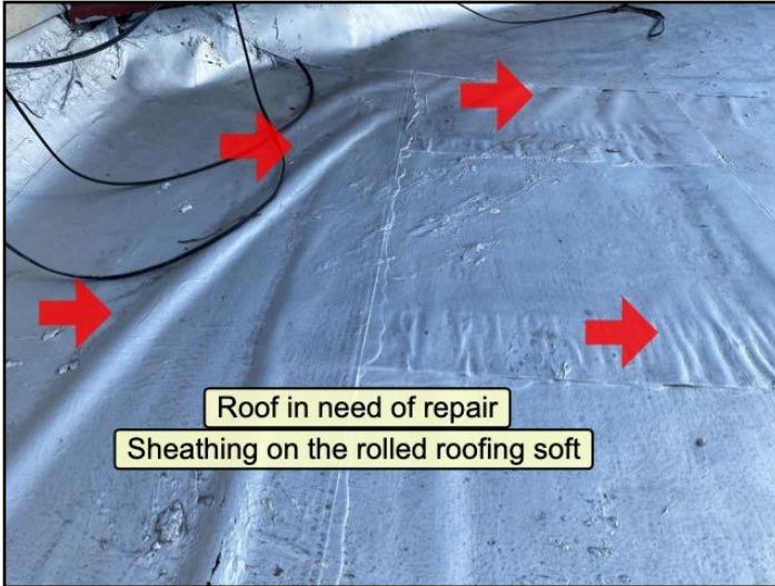
Licensed Roofing Contractor
