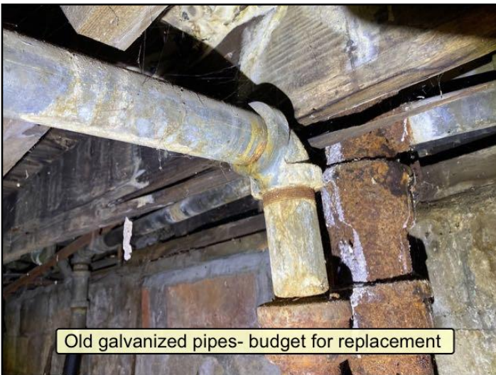
Old galvanized pipes rust from inside out...
