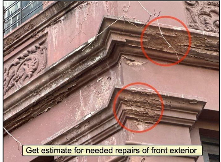
Masonry deterioration
