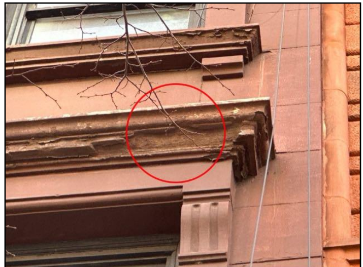
Masonry deterioration
