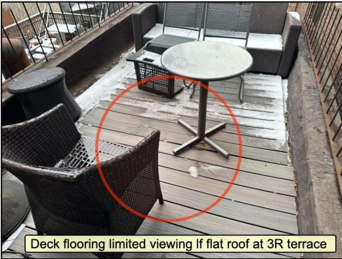
Deck covering roof
