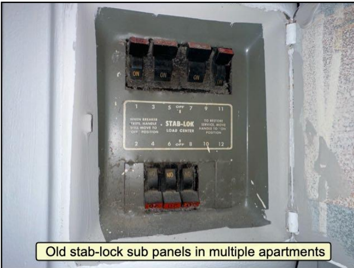
Old Stab-Lock panel and breakers
