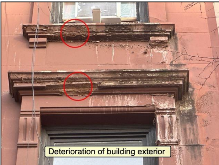
Masonry deterioration
