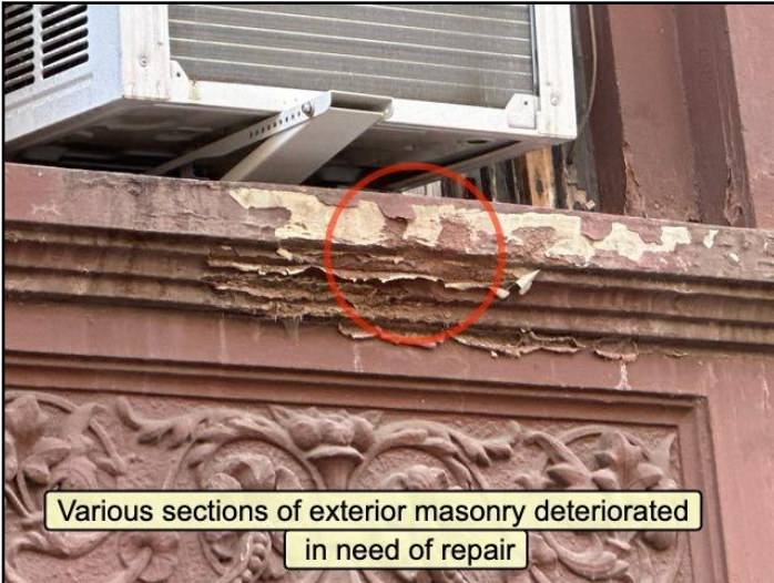
Masonry deterioration
