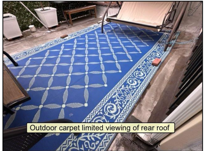
Deck covering roof
