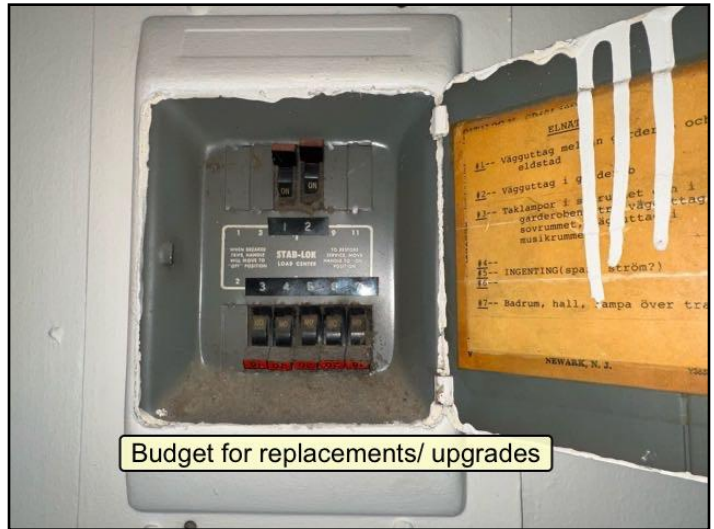
Old Stab-Lock panel and breakers
