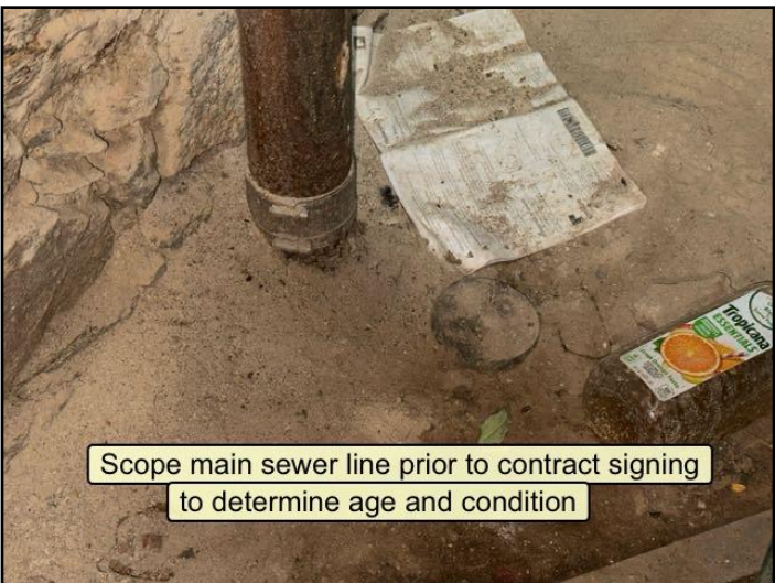
Scope main sewer line
