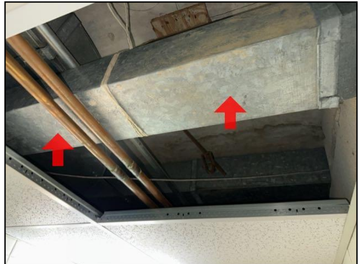
Older uninsulated ducts
