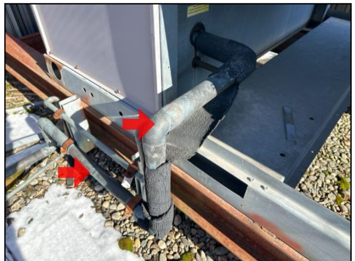
Insulation - missing
